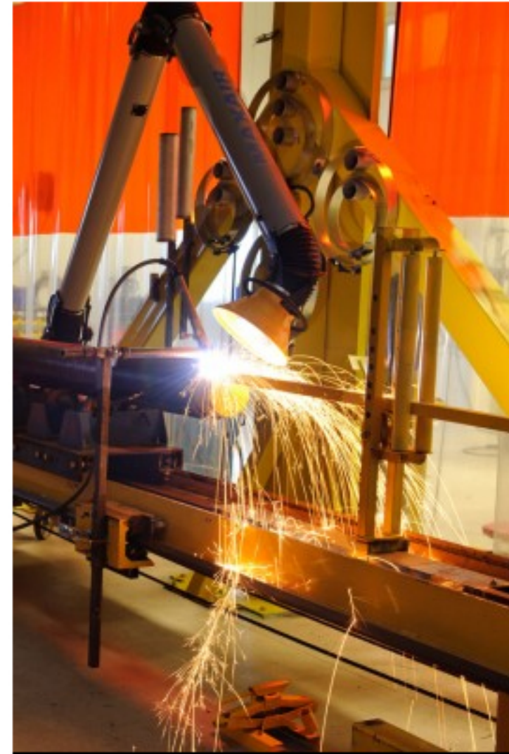
McNolty Mechanical uses plasma cutting equipment with automated rotation. It improves the accuracy and efficiency of the firm’s fabrication abilities in a competitive market.
